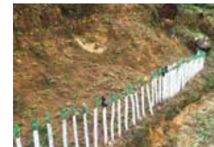
Soil runoff prevention fence
