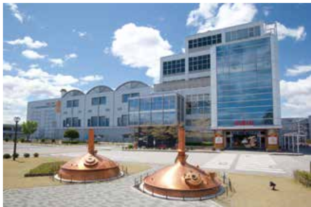
Kirin Brewery Nagoya Plant
