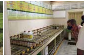
Chemical substance storage unit
