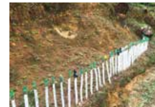
Soil runoff prevention fence
